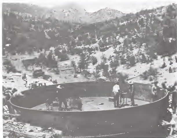
Figure 8. Cyanide leaching in large vats was used to recover gold from crushed ore. Photo courtesy Arizona Historical Society (AHS #72780).
